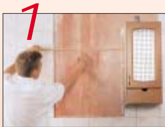
Measure the mirror and mark the area on the wall.
