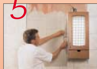
Put the connection tail of the mat into the flex pipe and push it up to the connection box.
