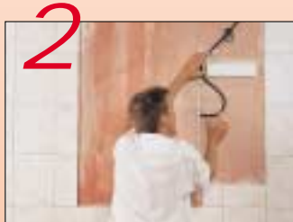
Mount a flex pipe in the wall from the mirror to the nearest connection box.
