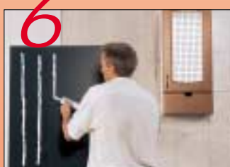
The mirror can now be mounted either directly in the tile adhesive or with acid free silicone after the tile adhesive has dried. Remember: the tile adhesive must be approved for mirror mounting.
