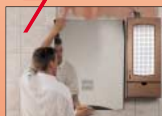
To improve the final look mount the tiles next to the mirror in line with it.
