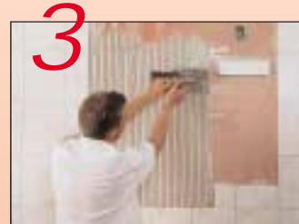
Cover the marked area with tile adhesive by using a toothed spatula. Remember to buy the sort of tile adhesive which does not attack the mirror – your local DIY store can help you.
